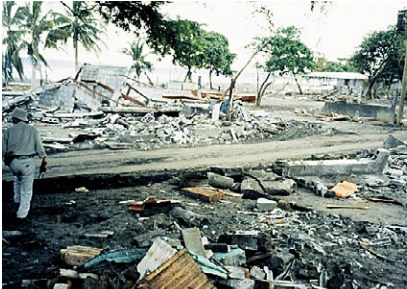
Damage from a tsunami
